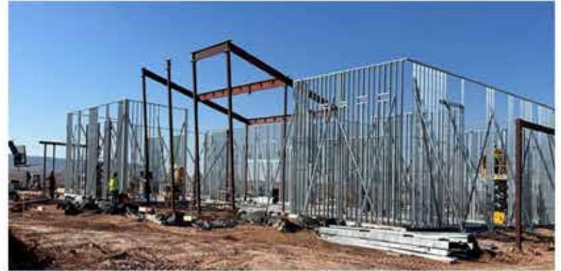
Red Mesa Sub-Office construction continues
