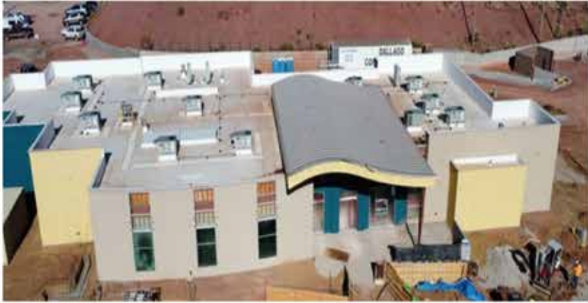
Construction progressing @ Fort Defiance District Office
