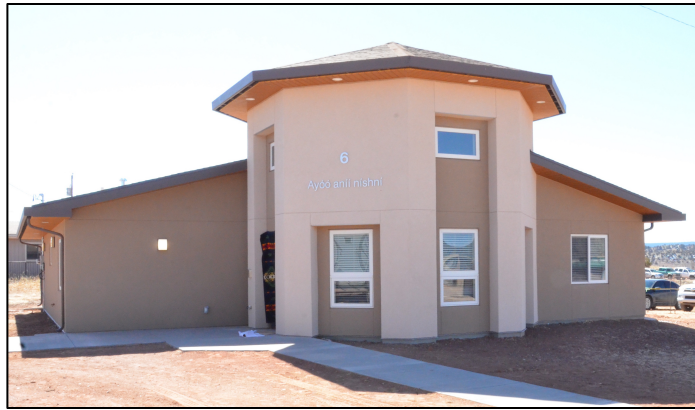
PHOTO: Newly constructed St. Michaels Association for Special Education group home.
